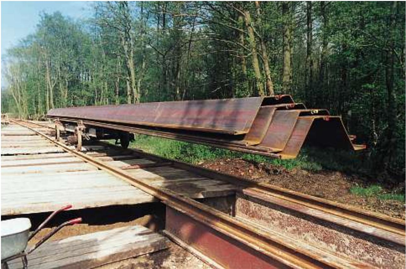
For this construction project, ProfilARBED supplied a total of 1,300 tonnes of 16 to 20.35 metres long AZ18 sheet piles.
