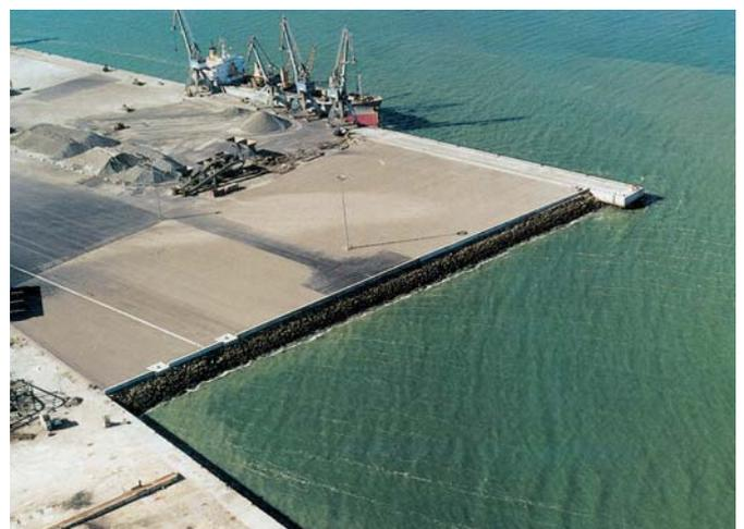
The quay extension required 1,600 metric tons of sheet piles
