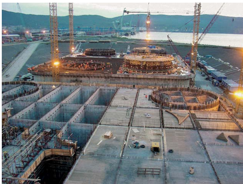
The 750-m outer dock wall features AU 25 and PU 32 piles
