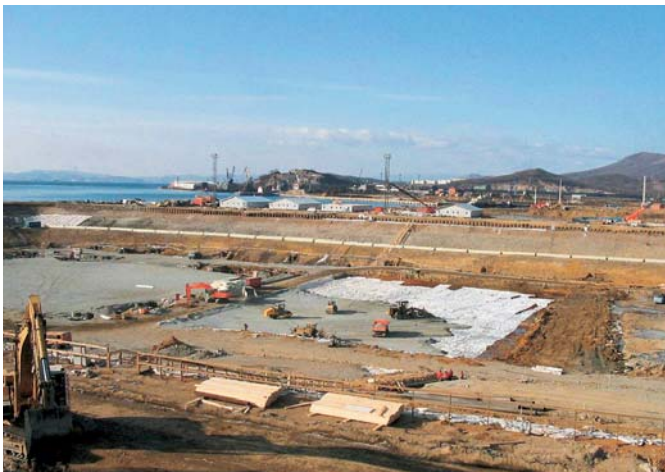
A dry dock for offshore platforms was built using more than 3,000 metric tons of steel sheet piles
