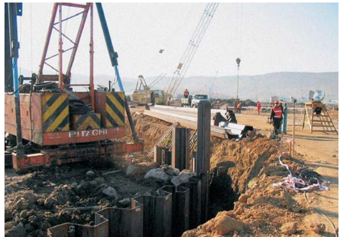
A dry dock for offshore platforms was built using more than 3,000 metric tons of steel sheet piles
