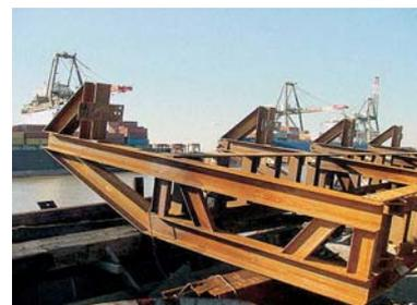
Neoprene shields attached to the template protected the coating system during installation
