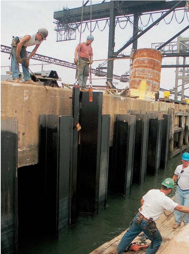
The heads of the HZ king piles remained above the water line, which facilitated their installation...
