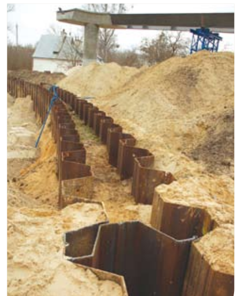
Steel sheet pile bridge abutment
