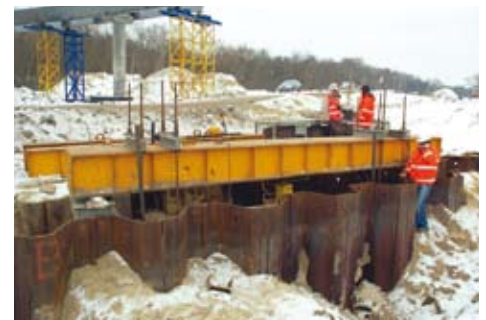
Static load test set-up
