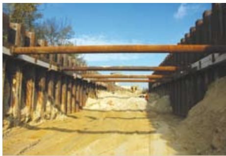
Construction phase of the underpass
