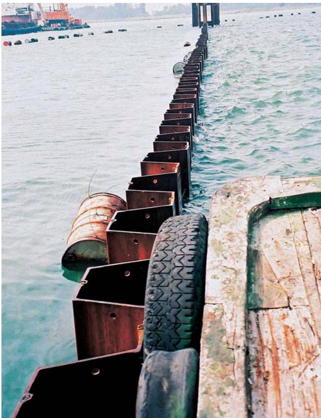
The installation team controlled the straightness of the wall axis optically
