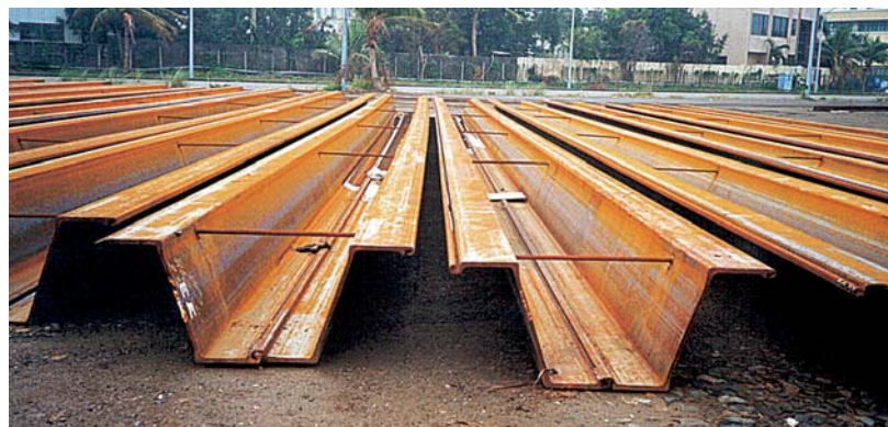
Welded on rebars prevent interlock rotation so as to precisely achieve the planned quay wall length
