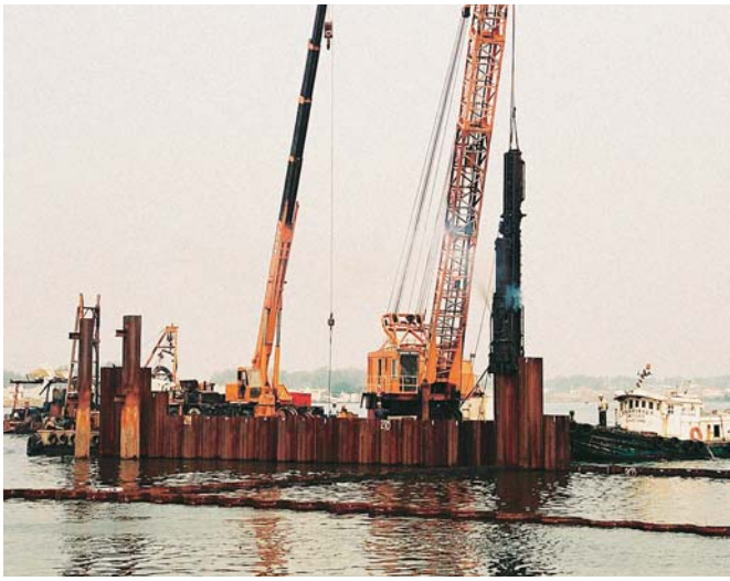
The sheet piles were installed in open water using barge-mounted vibratory and impact hammers
