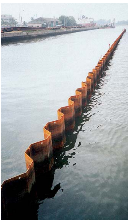
Anping Quay 1 - anchor wall
